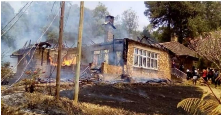
Figure 2: Hospital facilities torched by GDSFs in Kumbo
